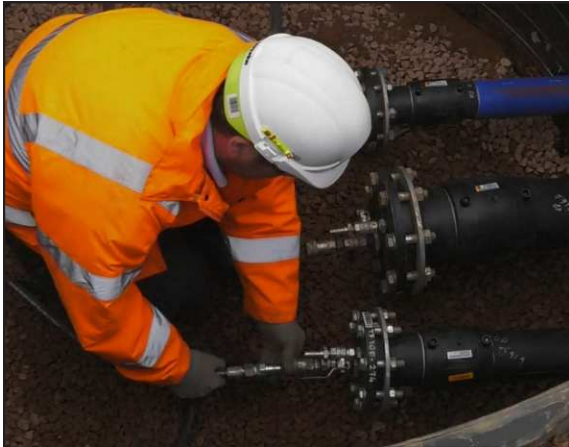
1. Connect the pump to the pipeline via the Valves and Pressure Test Box.
