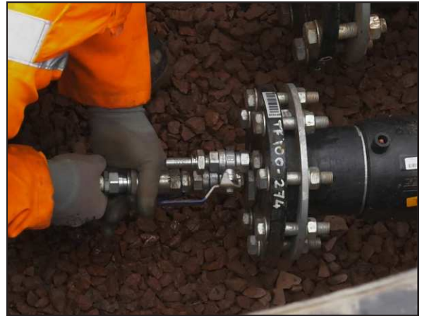
1. Connect the pump to the pipeline via the Valves and Pressure Test Box.
